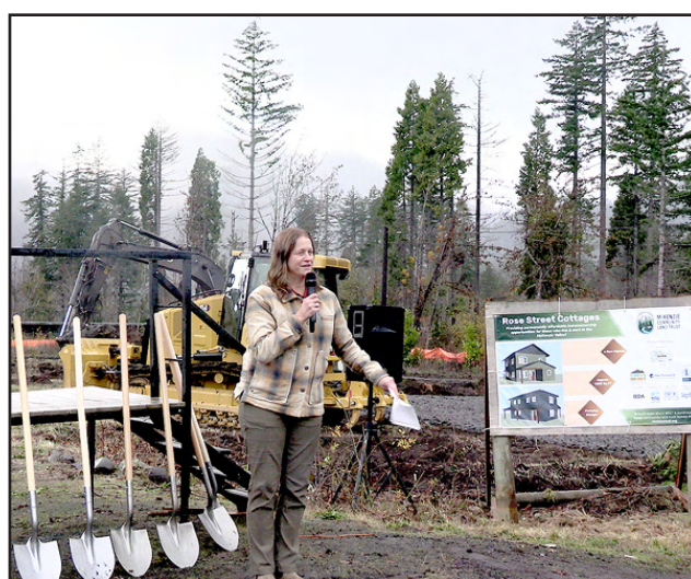
Shovels were at the ready on Friday for volunteers who dug up some small cedars for transplanting at the new Rose Street housing project site.
