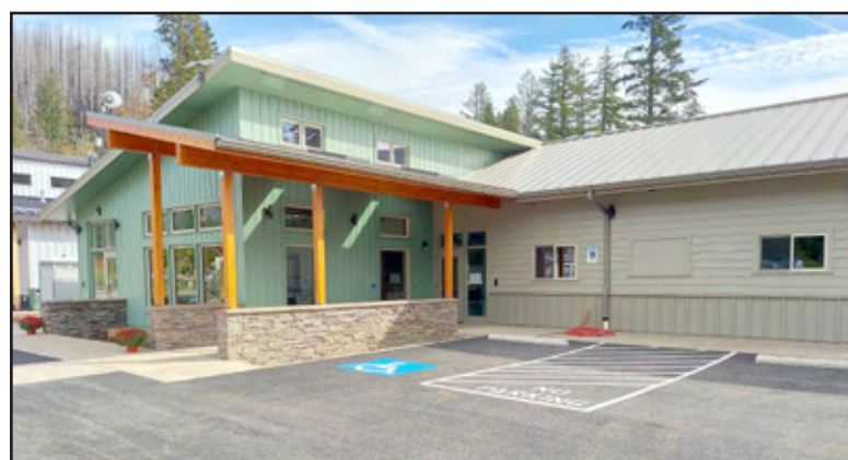
The new McKenzie River Clinic, next door to the Blue River Fire Station will open to the public on Friday.
