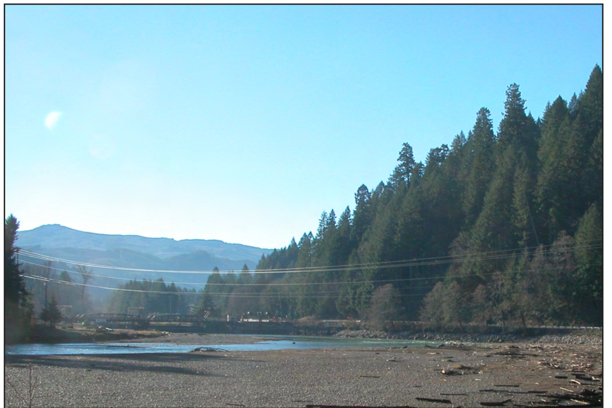
Property owners might lose lakeside frontage but gain additional mudflat acreage on the bottom of Leaburg Lake if the Eugene Water & Electric Board decides to remove the dam structure. What that could look like was apparent during a 2012 drawdown for rollgate repairs when the river channel shifted closer to the curve on Hwy. 126.
