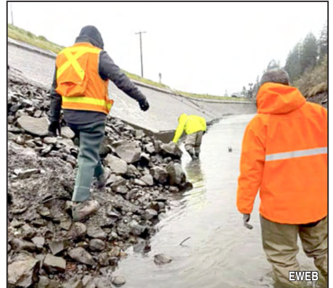
The Walterville Canal has been dewatered since February 27, 2024.
