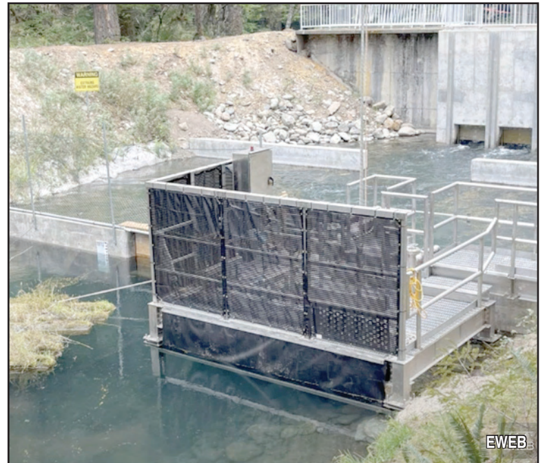
A temporary "catch and haul" system has been constructed to transport fish past the Trailbridge dam.
