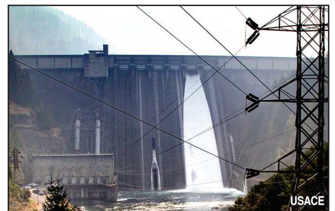
Detroit Dam southeast of Salem on the North Santiam River provides hydropower and flood risk management but also blocks fish passage.
